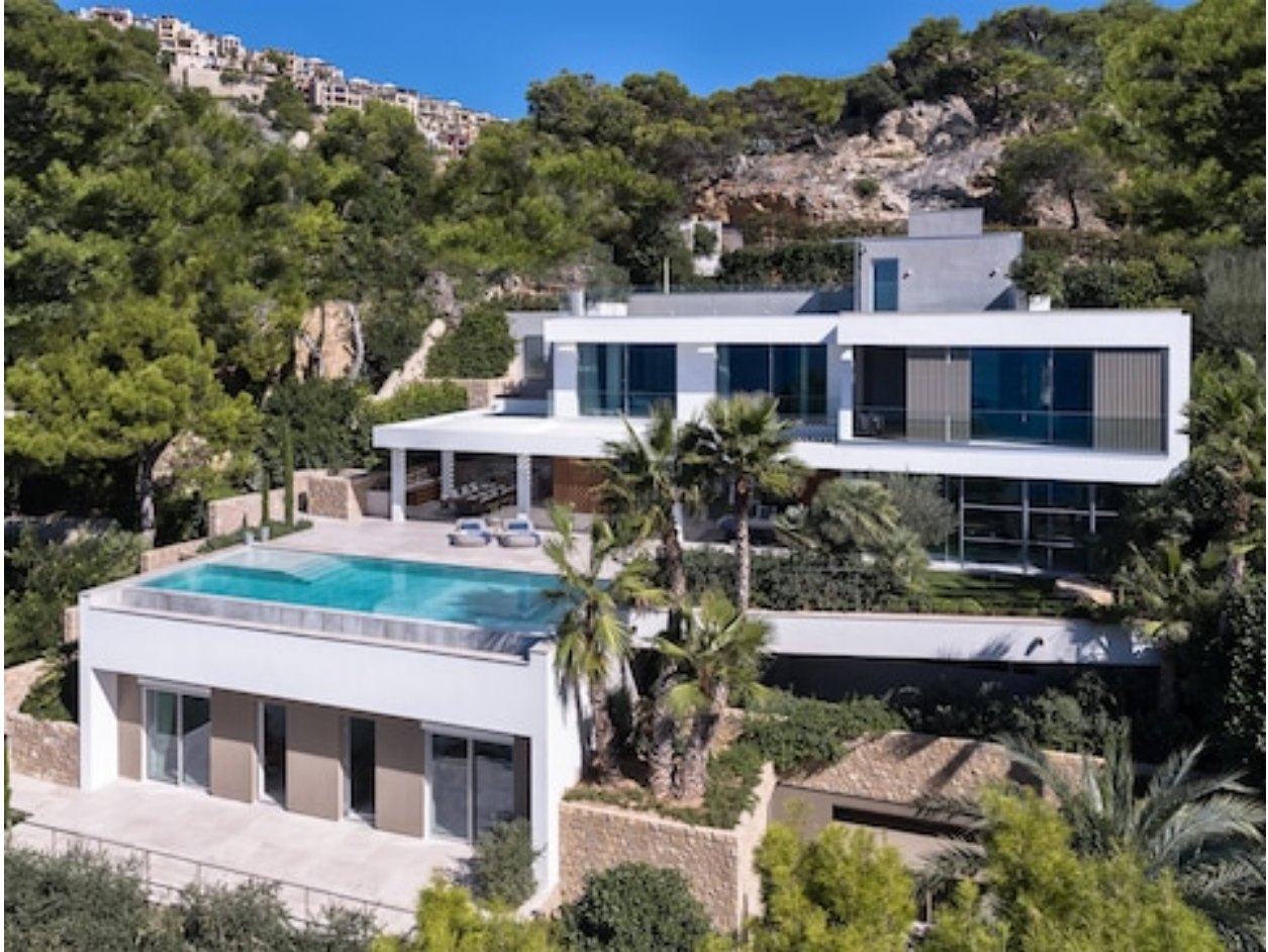
The Seahouse in Puerto Andratx, Mallorca
